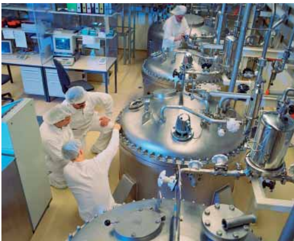
Downstream: Buffer preparation.
